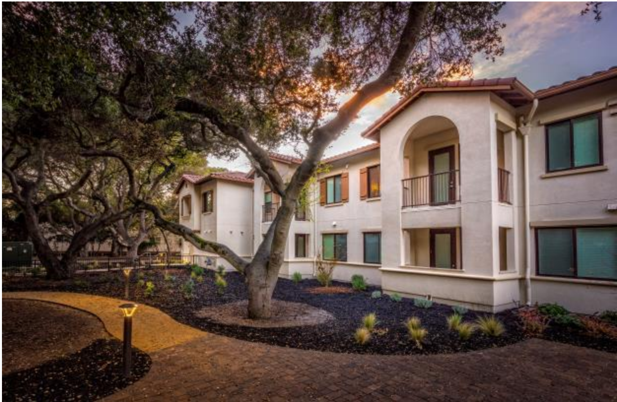
Figure II-2: Actual VA EUL Permanent Supportive Housing Facility
