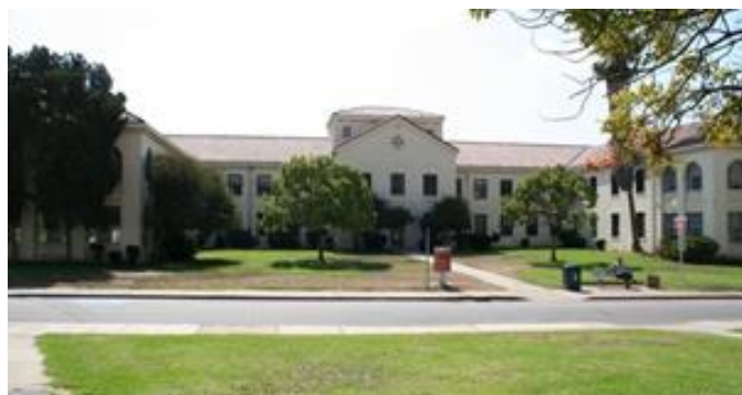
North Campus, Subarea 4, Neuropsychiatric Hospital, Building 258, constructed 1946, view northwest (VA Archives, circa 1950s).
