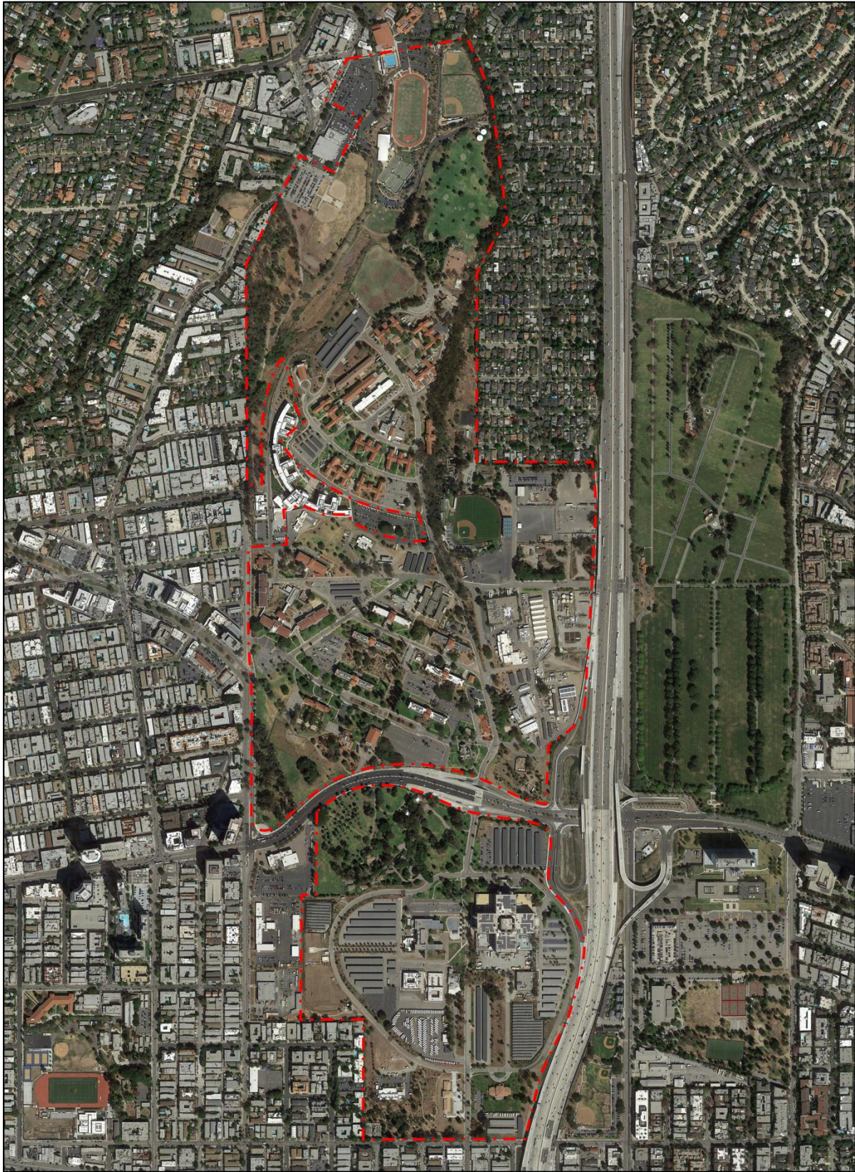
Figure V-1: Aerial View of Existing Campus
