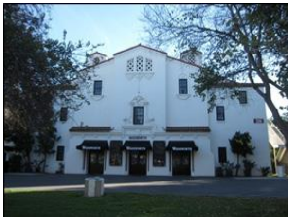
North Campus, Subarea 1: Bldg. 66, News Stand (Streetcar Depot), constructed 1890.
