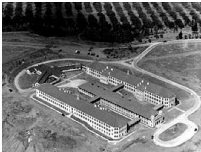
North Campus Subarea 4: Neuropsychiatric Hospital area, Buildings 156, 157, 158, constructed 1923 (n.d.), north perspective.
