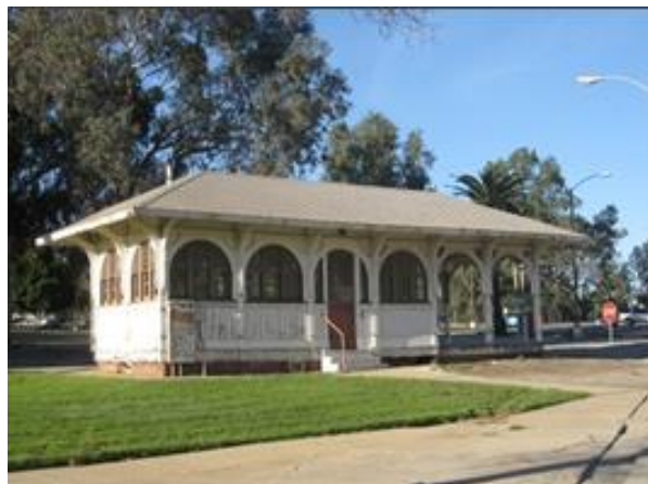
North Campus, Subarea 1: Building 226 (Wadsworth Theater), constructed 1940, north elevation
