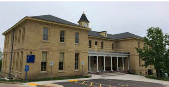
Old Administration Building
