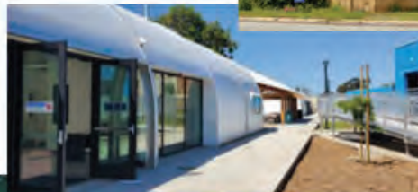
Emergency Housing: e.g., A Bridge Home (ABH) Shelter
