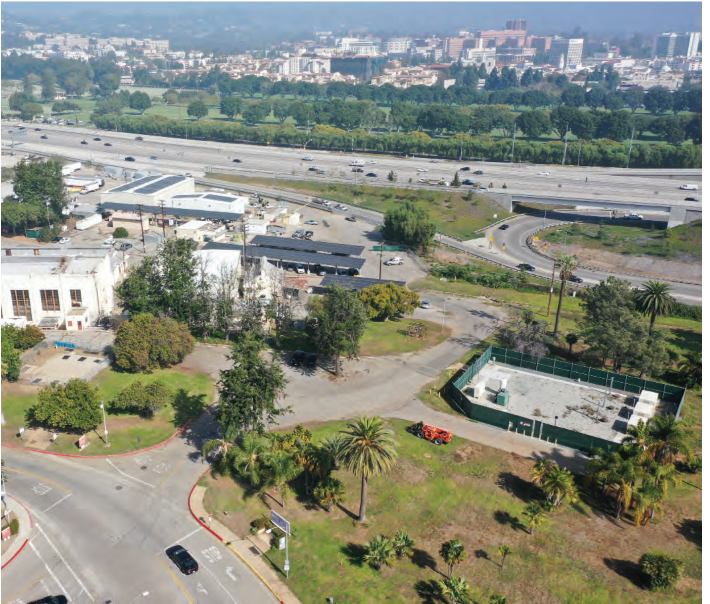
A view to the east, showing the knoll and southern portion of the Auxiliary Services Area, which could be considered for job training uses
