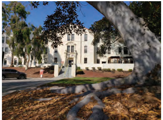
View of Building 215 in Zone 2
