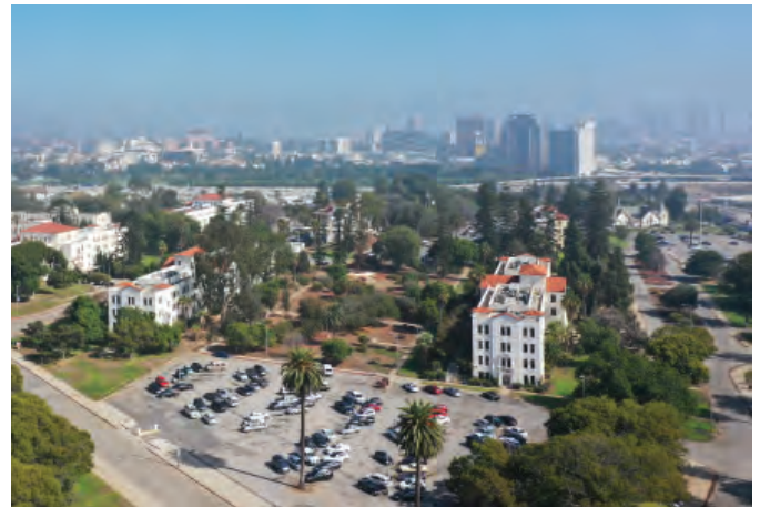
A view to the east with Buildings 214 and 217 in the foreground
