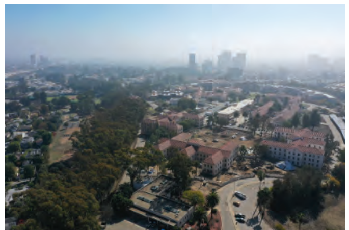
Aerial view of the Campus looking south - steep bluffs on the eastern edge
