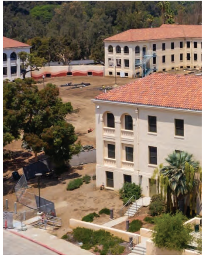
Buildings 205 & 208 - 122 units (Under Construction)
