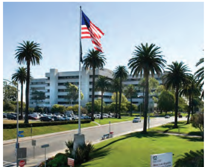
Building 500 is anticipated to be renovated in the Interim Phase
