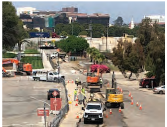
Bonsall Utility Trunk Line Under Construction
