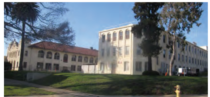
Building 158, Flex Space
