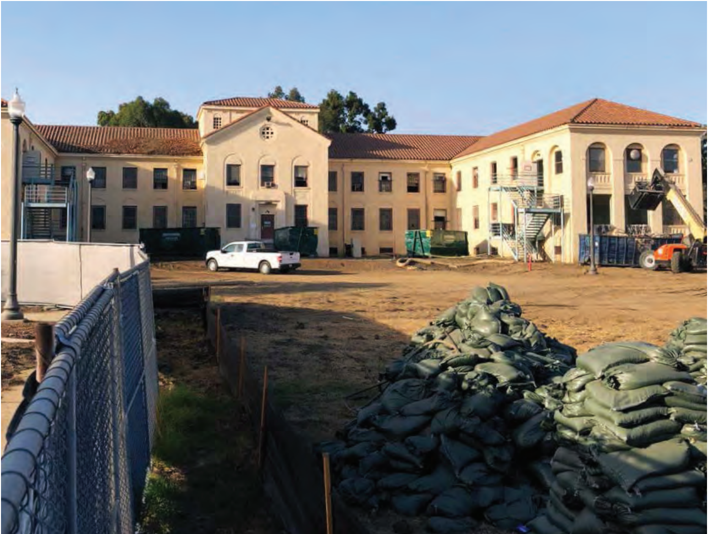
EUL Housing Under Construction (Building 208)
