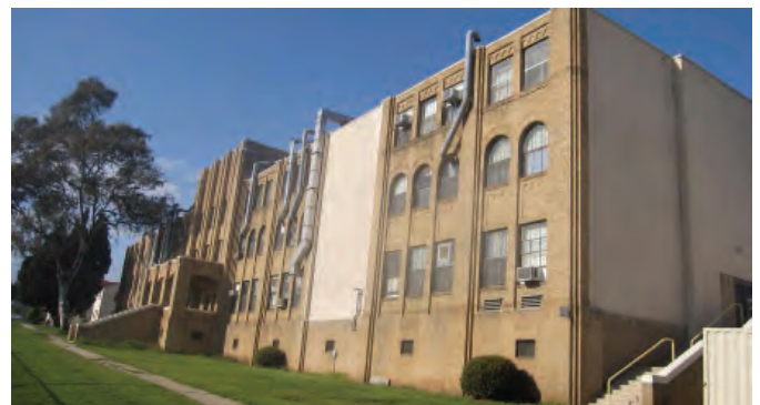
Building 115, Research Building
