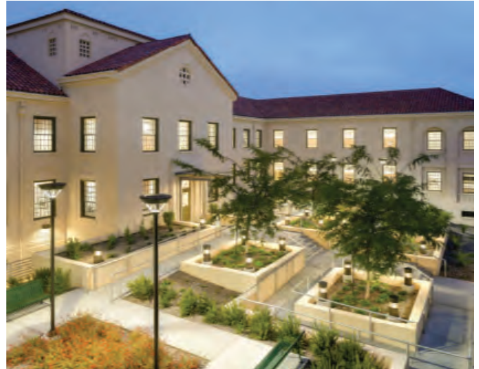
EUL Housing in Building 209
