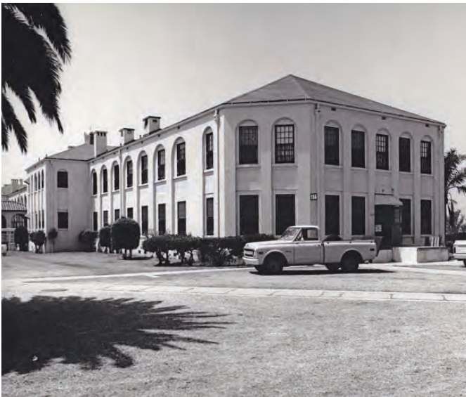
Building 156 (extant), view southwest (VA Archives, circa 1972)
