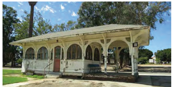
Building 66, Historic Trolley Depot, individually listed in the National Register of Historic Places
