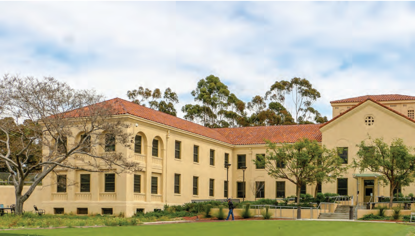
Building 209, West LA Campus
