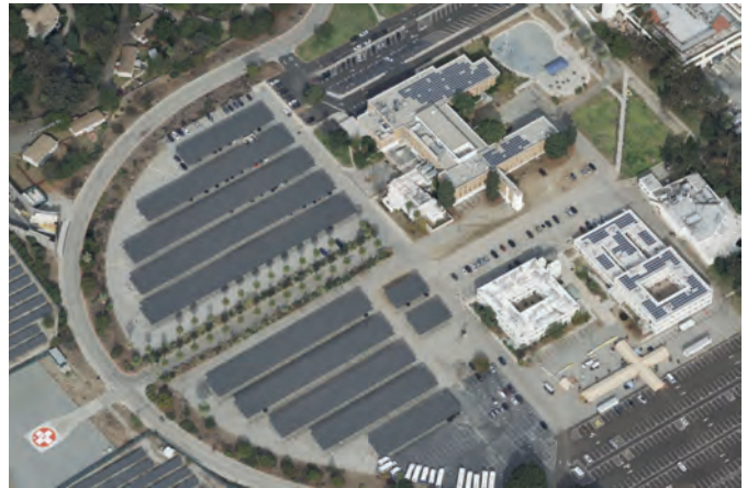
Solar panels on the parking lots and roofs of building 304 and 401 in the South Campus
