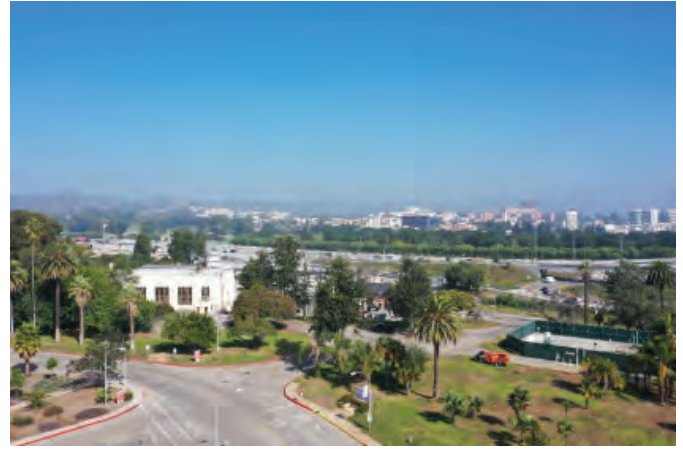
A view to the northeast of Building 295 and the Auxiliary Services Area
