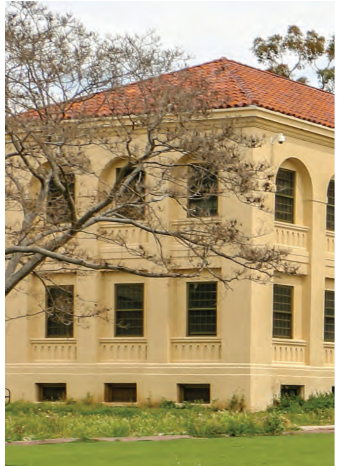
Building 209, West LA Campus
