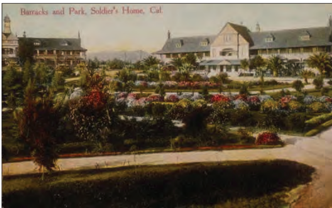
Domiciliary, Barracks #4 (left, not extant) and #5 (right, not extant), view northeast (Santa Monica Public Library, 1890)
