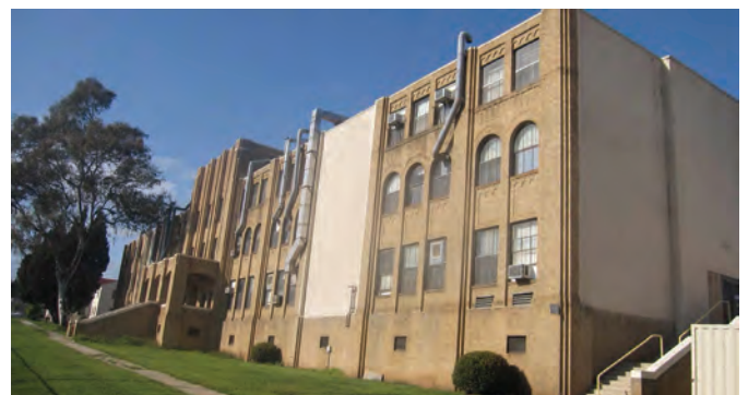
Building 115, Research Building
