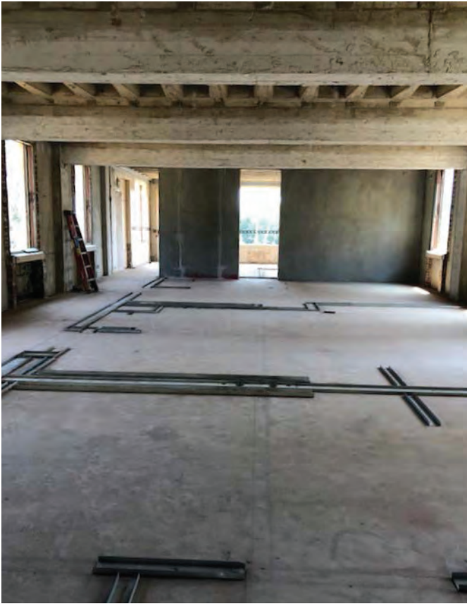
Building 207 - 60 units (Under Construction)
