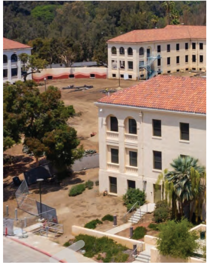
Buildings 205 & 208 - 122 units (Under Construction)
