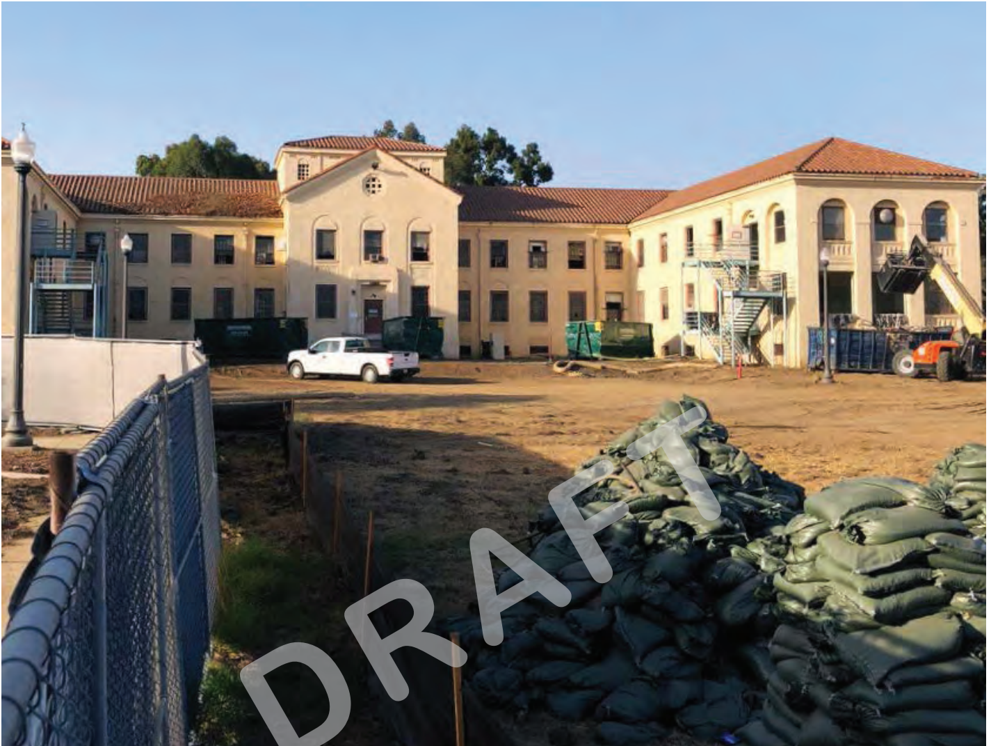
EUL Housing Under Construction
