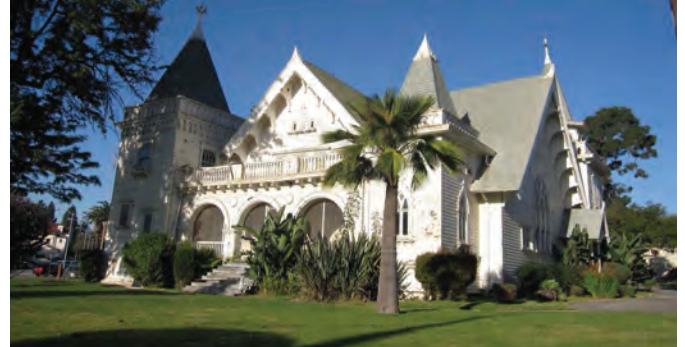
Building 20, Wadsworth Chapel
