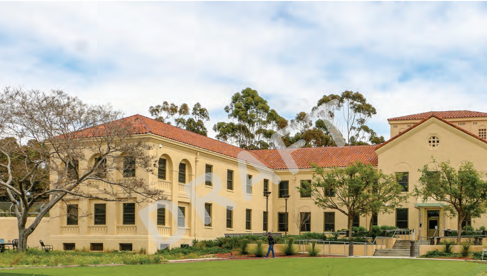
BUILDING 209, WLA CAMPUS
