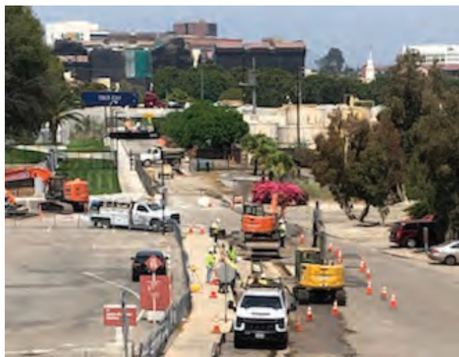
Bonsall Utility Trunk Line Under Construction
