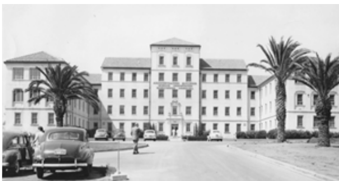
Northwest Quadrant, Subarea 4, Neuropsychiatric Hospital, Building 258, view northwest (VA Archives, circa 1950s).
