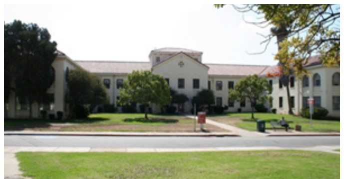
Northwest Quadrant, Subarea 4, Neuropsychiatric Hospital, Building 256, constructed 1946. North elevation.
