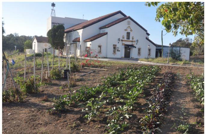
Building 211 - Brentwood Theater
