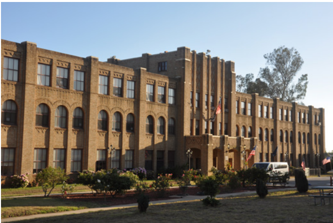
Building 116 - New Directions
