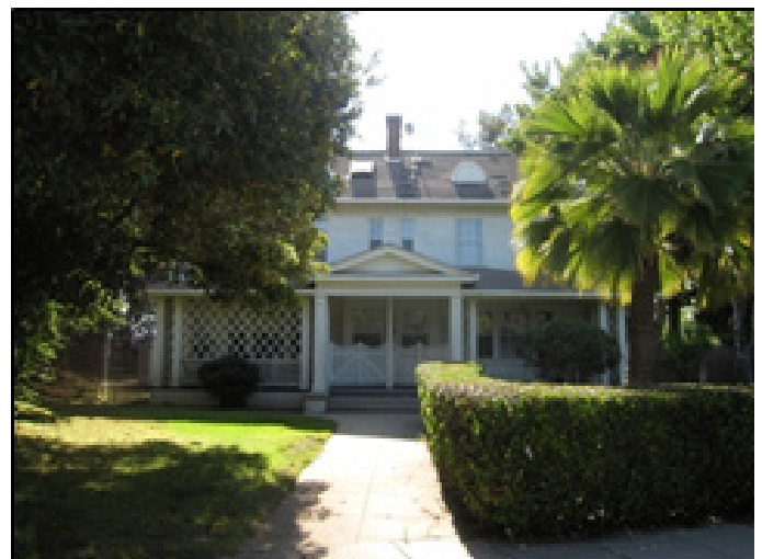
Northwest Quadrant, Subarea 2, Building 90, constructed 1927 (altered 1995). West elevation.
