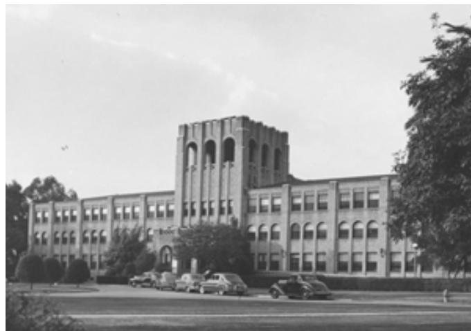
Northwest Quadrant, Subarea 3: Research, Building 114, view northeast (VA Archives, nd).
