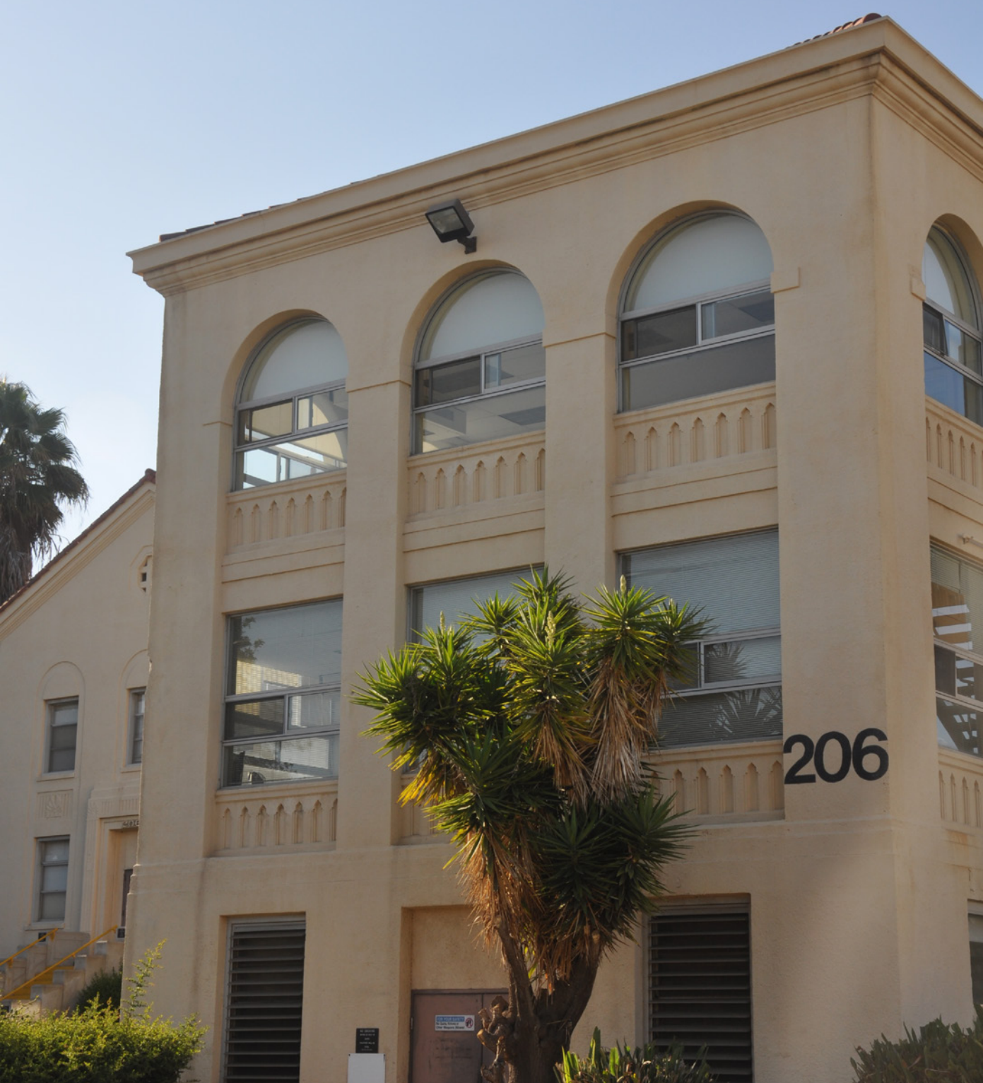
Building Numbering, Building 206
