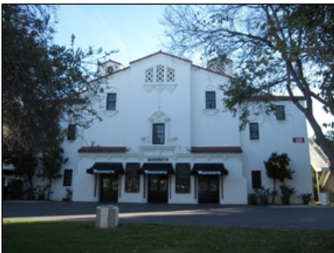
Northwest Quadrant, Subarea 1: Building 226 (Wadsworth Theater), north elevation
