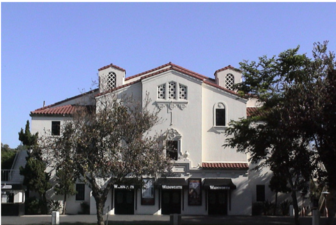
Building 226 - Wadsworth Theater
