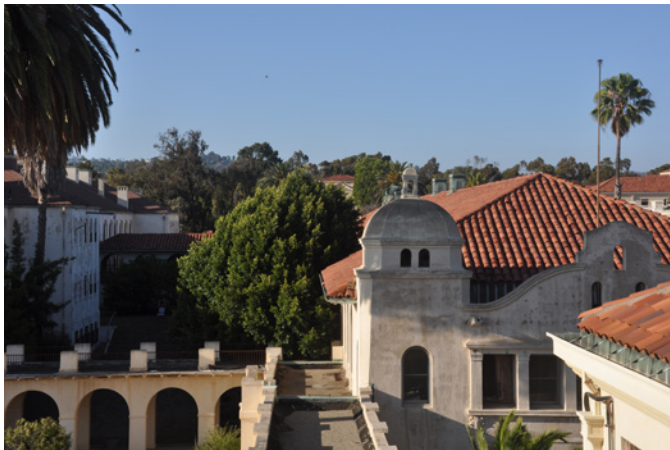
Existing Building Roofscape, Building 157
