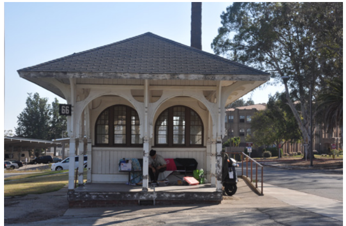
Building 66 - Trolley Depot
