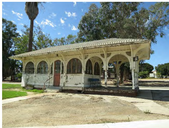
Figure 3.3-7. Streetcar Depot (Building 66), September 2017
