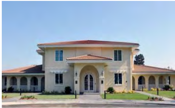
Figure 3.1-11. Fisher House (Building 523)
