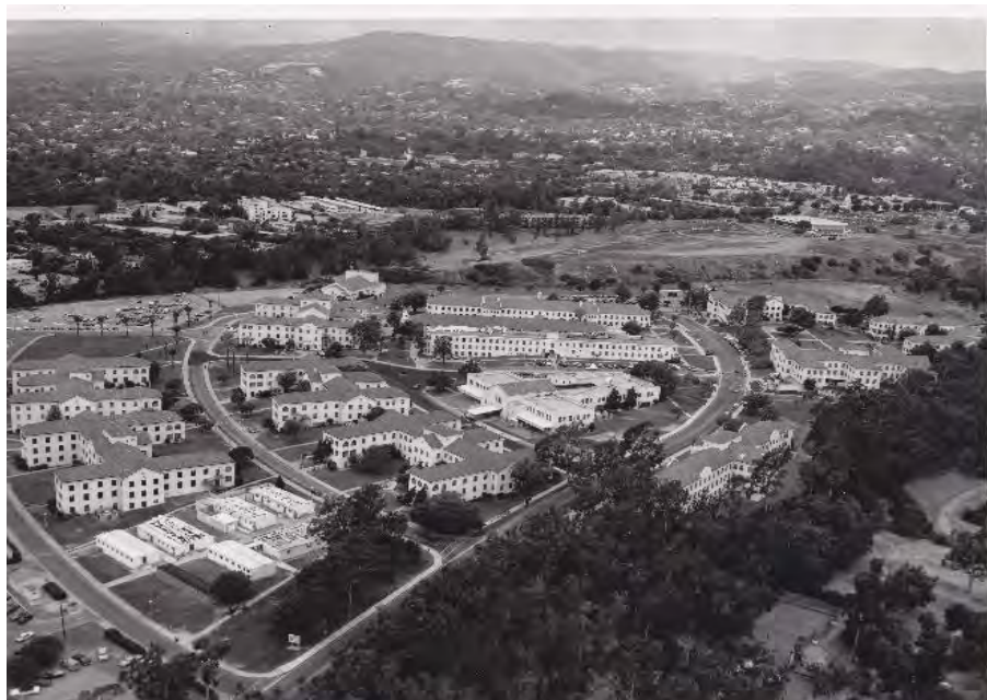
Figure 3.3-2. Aerial Image of the WLA Campus (August 1984)
