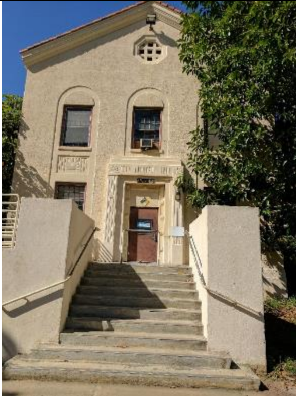
Building 208 entrance (south side facing courtyard)
