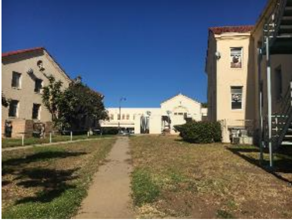
West side of Building 207 (right side of photo), south side of Building 300 (center of photo in background), and east side of Building 206 (left side of photo)
