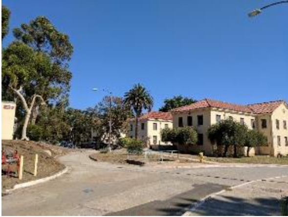
Building 208 from north side
