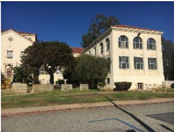
Southeast side of Building 207
