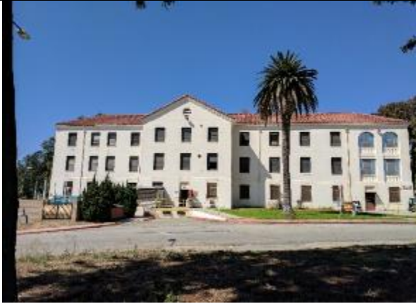
South side view of Building 205 (courtyard and Parking Lot No. 27 are east of building)
