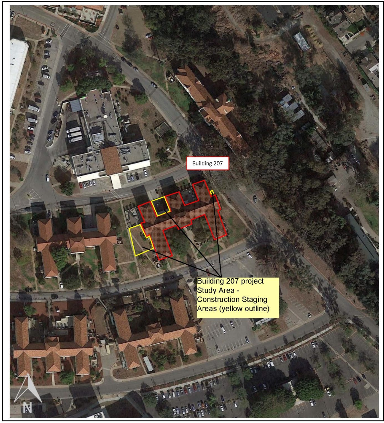
Figure 4. Building 207 Project Study Area - Construction Staging Area
