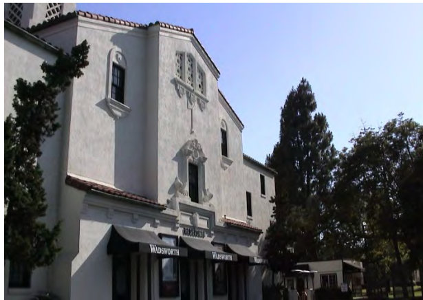
Wadsworth Theatre (Building 226)
