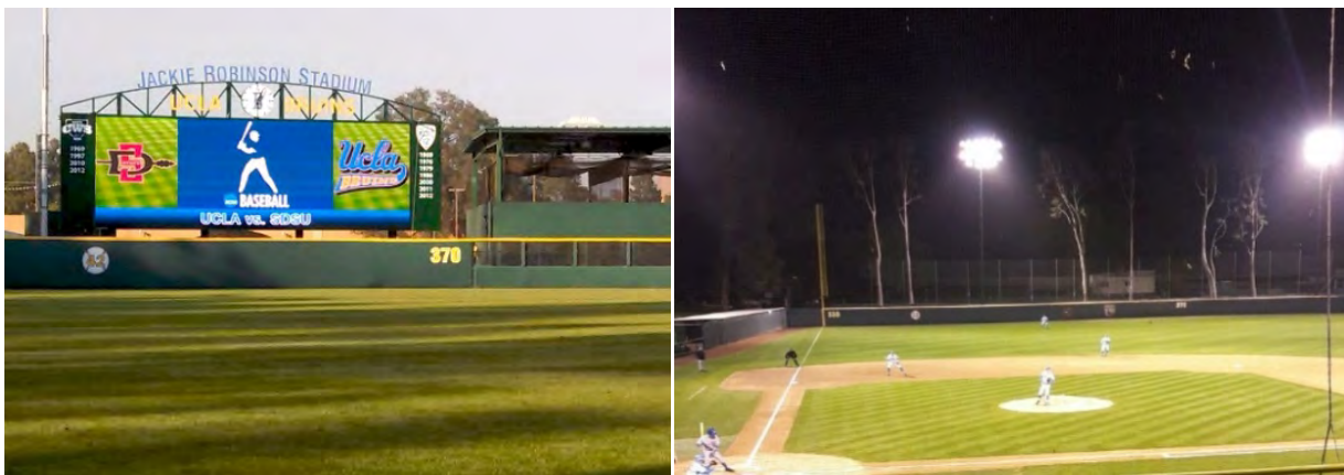
Figure 3.1-13. Jackie Robinson Stadium Lighting and Video Scoreboard
