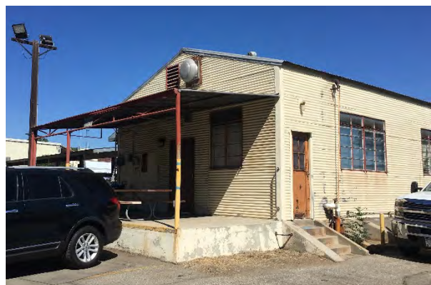
Transportation Offices (Building 305)
