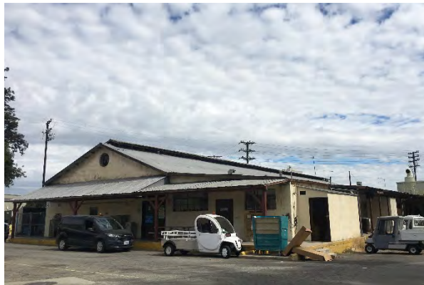
Plumbing Shop (Building 46)
