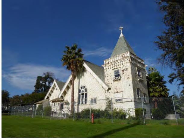
Wadsworth Chapel (Building 20, NRHP-Listed)
