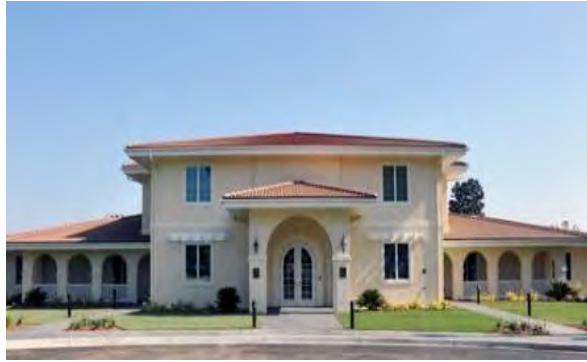
Figure 3.1-11. Fisher House (Building 523)
