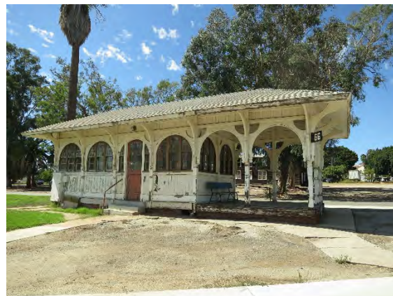
Figure 3.3-7. Streetcar Depot (Building 66), September 2017
